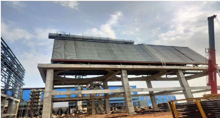
Air Cooled Condenser
